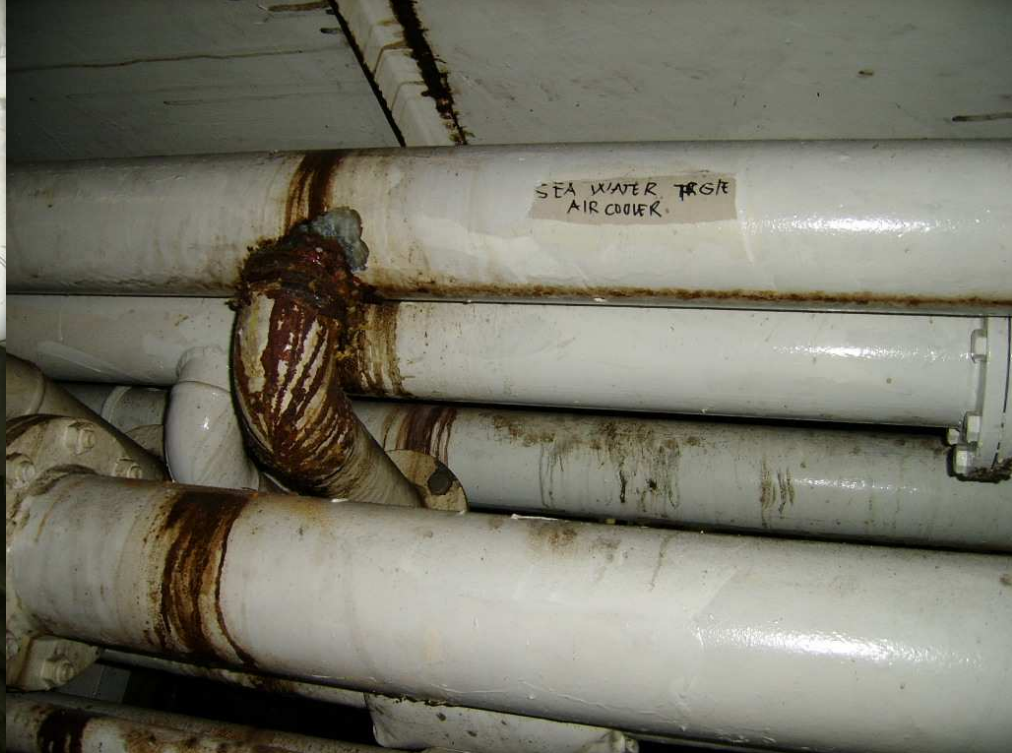
MV Caribbean Mermaid: Numerous temporary repairs at important piping systems in the engine room
